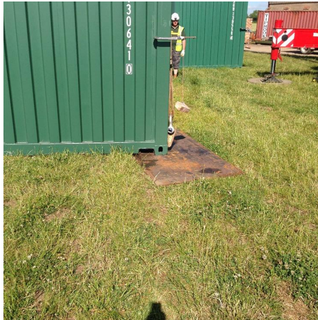
Figure 2. Containers leveled using steel plates
