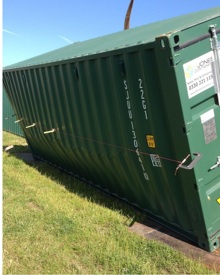
Figure 6. Failure of side wall panel. Measurement points shown
